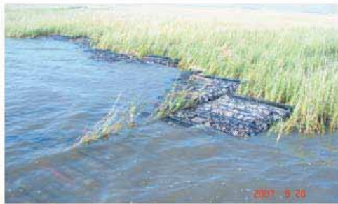
Installed Gabion Mats along the north shore of Lake Barre.
