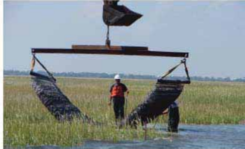
Installation of Gabion Mats (one of the three techniques being used on this project) along the north shore of Lake Barre.
